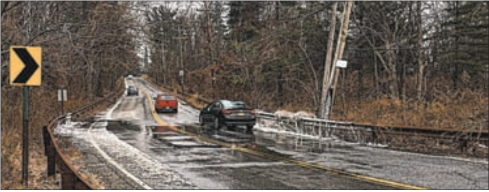
Icy road conditions are caused by water flowing across Shore Road.
