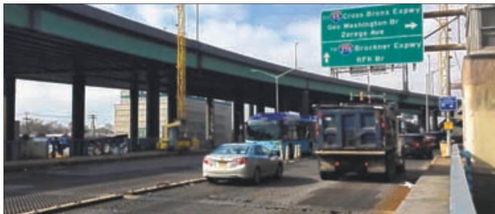
Work begins on a four-year reconstruction project on the Unionport Bridge over Westchester Creek on or around Thursday, February 22. Community News Group / Patrick Rocchio
