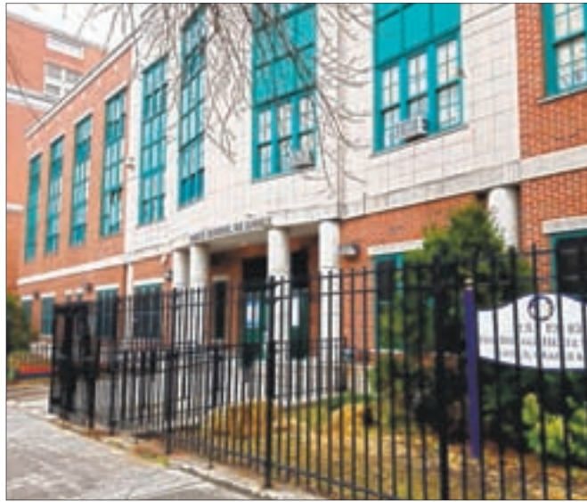
The P.S. 83 Annex is among the buildings in the Bronx found to have elevated lead levels in its water pipes. The water systems are being remediated, according to the NYC Department of Education.
