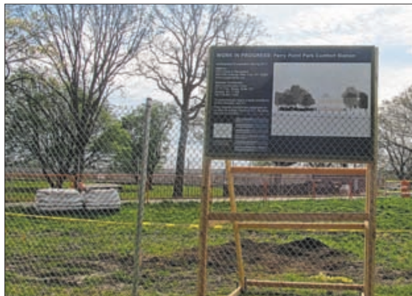
A sign tells parkgoers of a ‘work in progress,’ a comfort station budgeted close to ten years ago.
