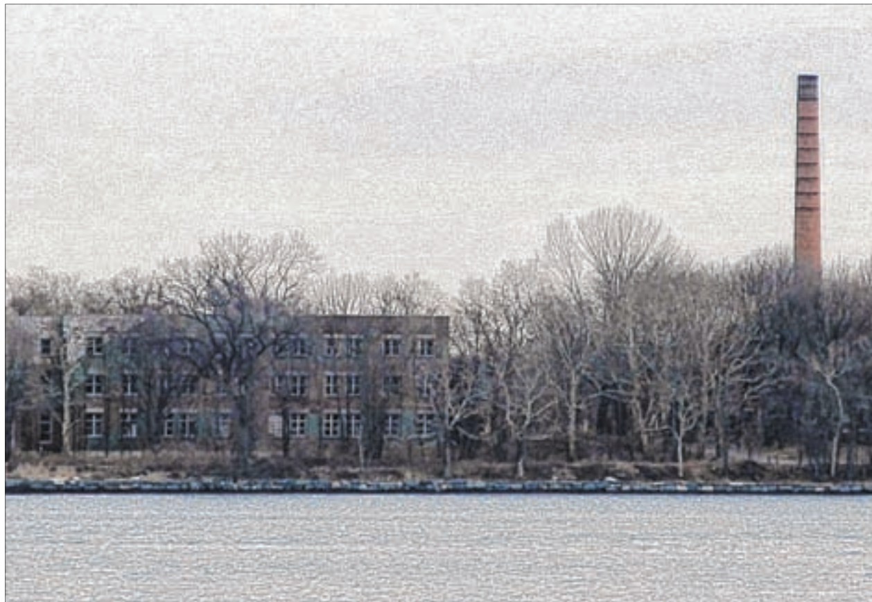
The Parks Department expressed skepticism about transferring it jurisdiction of Hart Island.
