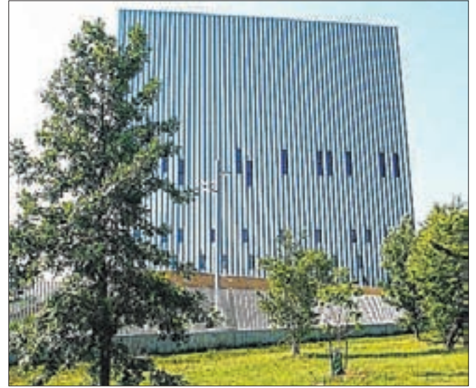
The Public Safety Answering Center II located at 350 Marconi Street, as seen from the Hutchinson River Parkway. Photo by Walter Pofeldt
