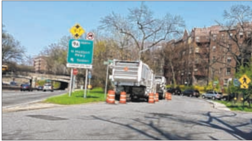
Construction vehicles mobilize on the Henry Hudson Parkway in the Bronx to begin renovations. Photo by Miriam Quin
