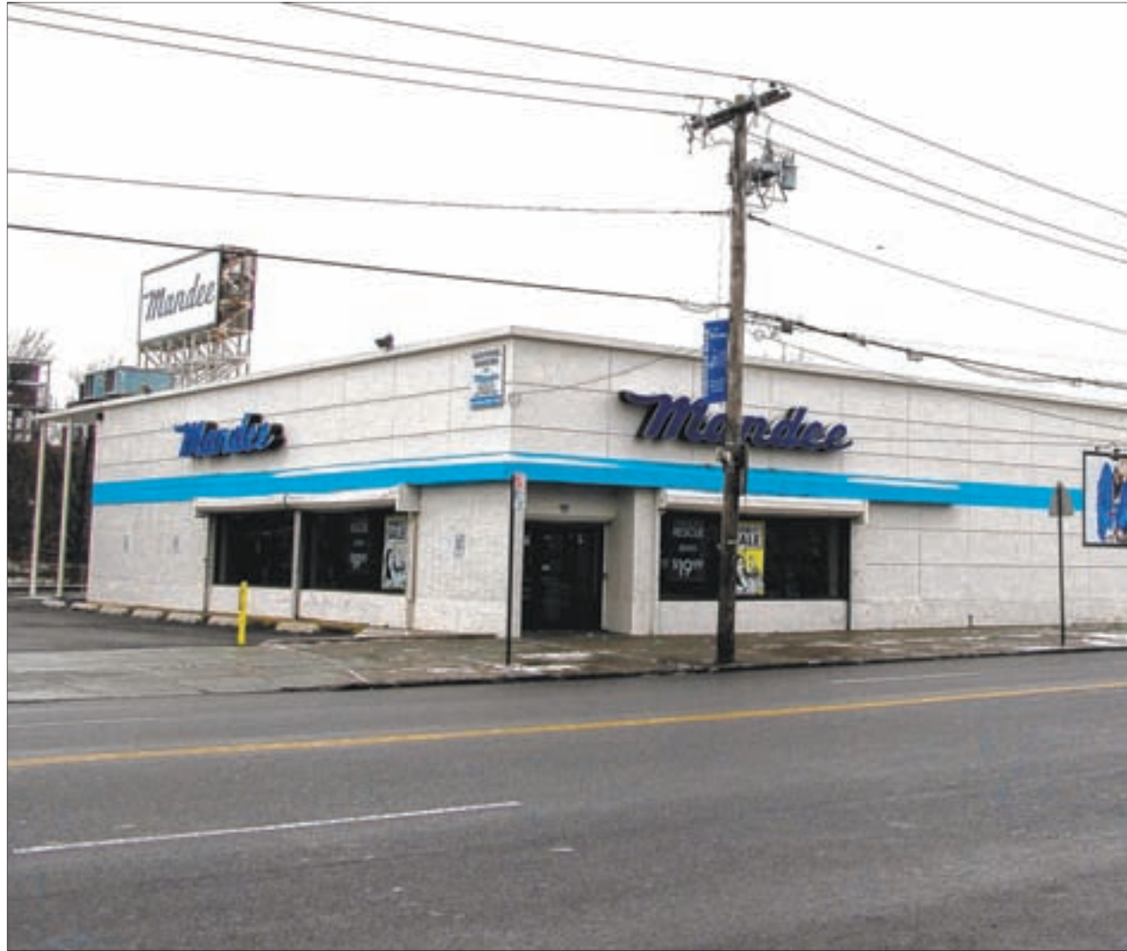
The E. Tremont Avenue property which once housed Mandee is being pushed by community leaders to become the next home to the 45th Precinct and Police Service Area #8.
