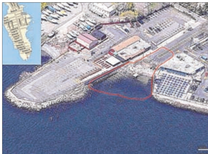
A Parks Department bird's eye view of the site where the park is going to be constructed is seen here. The park area is circled in red. Photo courtesy of the Parks Department
