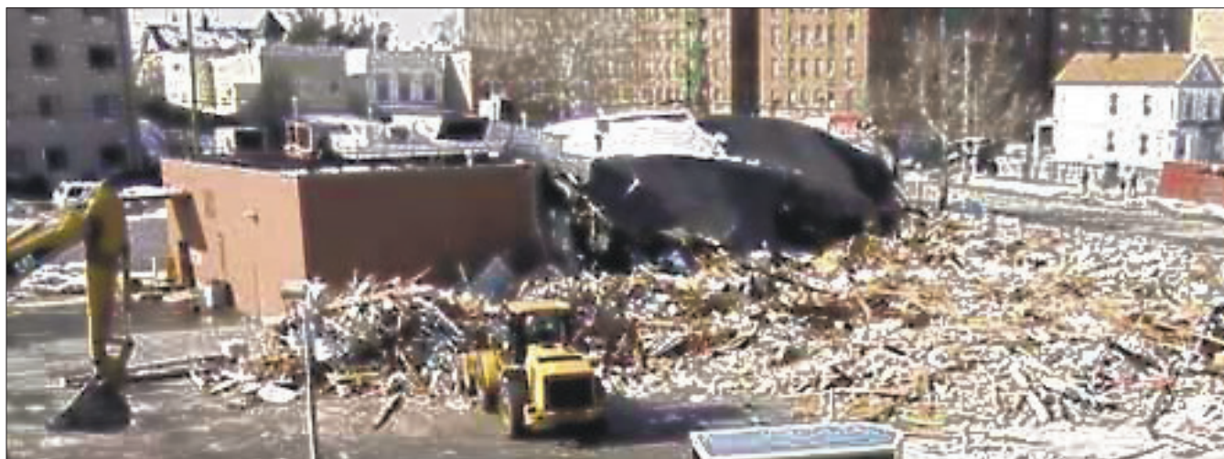
The CVS at Burke Avenue and White Plains Road was demolished after the roof collapsed in February 2014. CVS is rebuilding and plans to reopen the location this summer.
