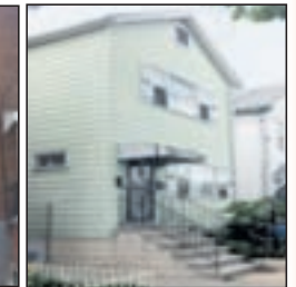
2 Family. Income Basement apartment and 2 car garage. $490,000.
