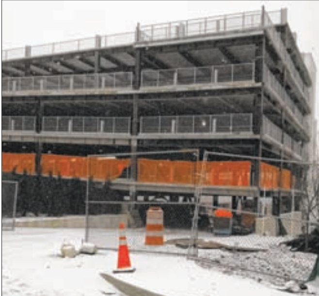
The west parking garage, located on Bassett Avenue, will be the second parking garage within Hutchinson Metro Center.
