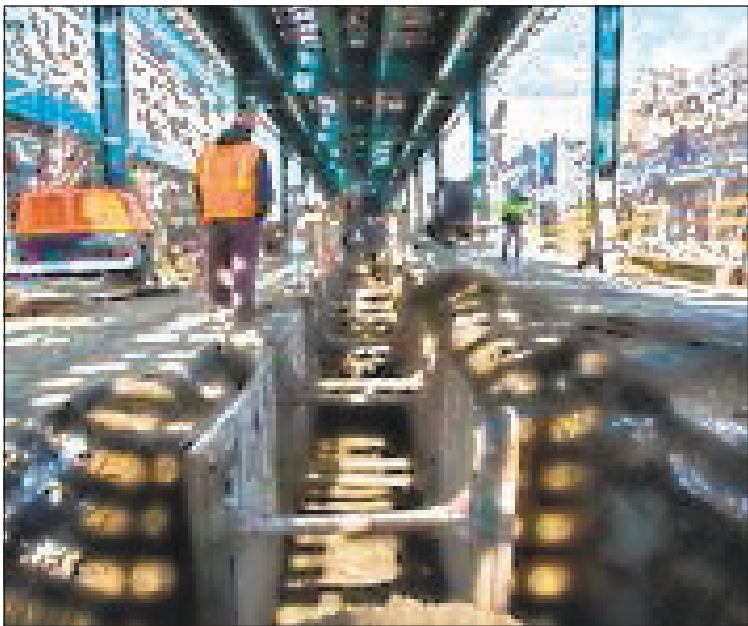
Construction workers installing sewer upgrades along Southern Boulevard. Photo Courtesy of the New York City Department of Design and Construction
