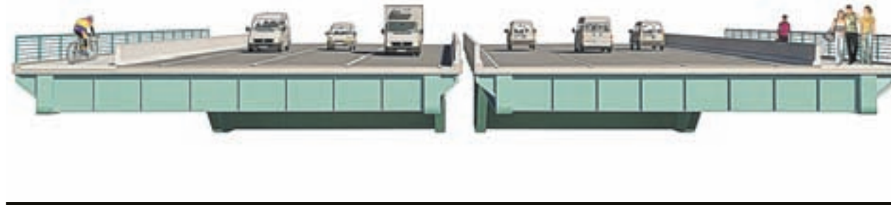
An artist rendering of the replacement Unionport Bridge that features three lanes in each direction and dedicated bicycle/pedestrian passages. Photo courtesy of DOT
