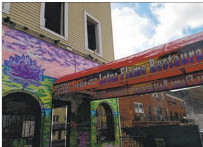
The Lotus Flame restaurant in Morris Park is closed indefinitely due to a fire that occurred last week. A family living in an apartment above was also displaced. Arthur Cusano
