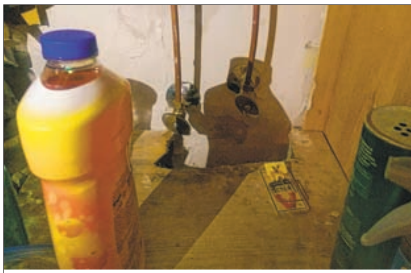
A hole under the sink was left by plumbers in one of the Woodmansten apartments
