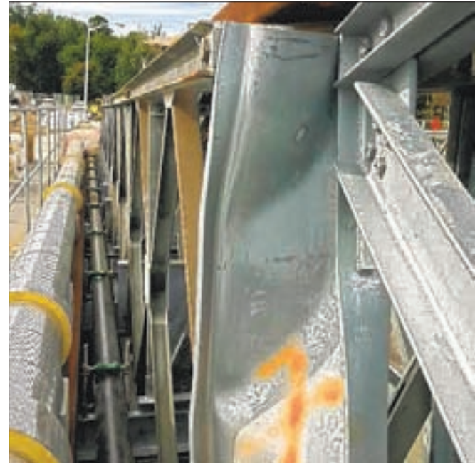
This photo, submitted to the Bronx Times, shows some of the damage caused to the temporary causeway bridge under construction. The bridge is located next to the existing City Island Bridge and suffered a failure when part of its roadway collapsed during its paving several weeks ago.
